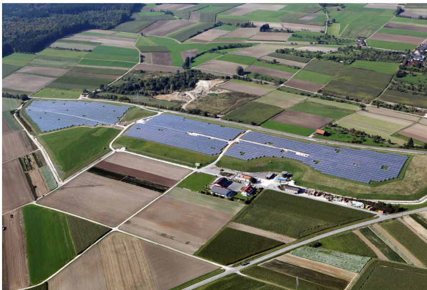
Solarpark Deponie Eggingen
